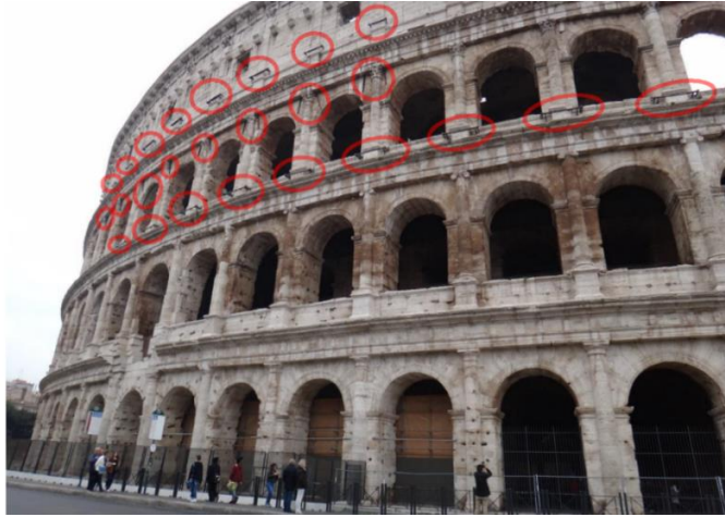
Figure 2c. Fasteners by Canina for 60 Cm out plumb (1830-1850).
