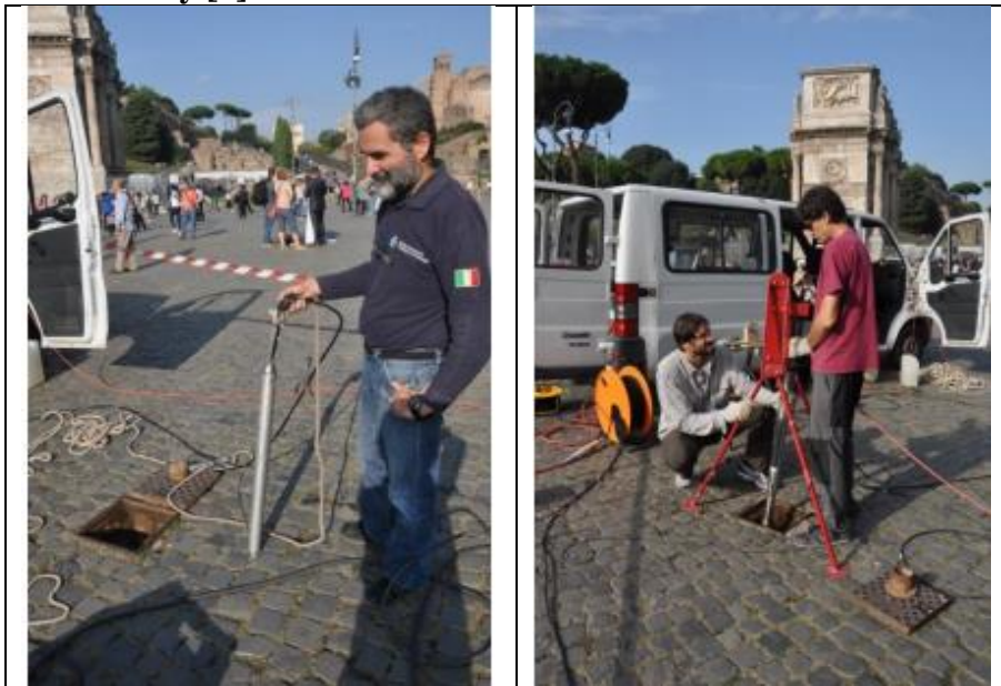
Figure 11. Inserting in existing boreholes (up to 47 m) of: Geophone in A); sparker source in B)
